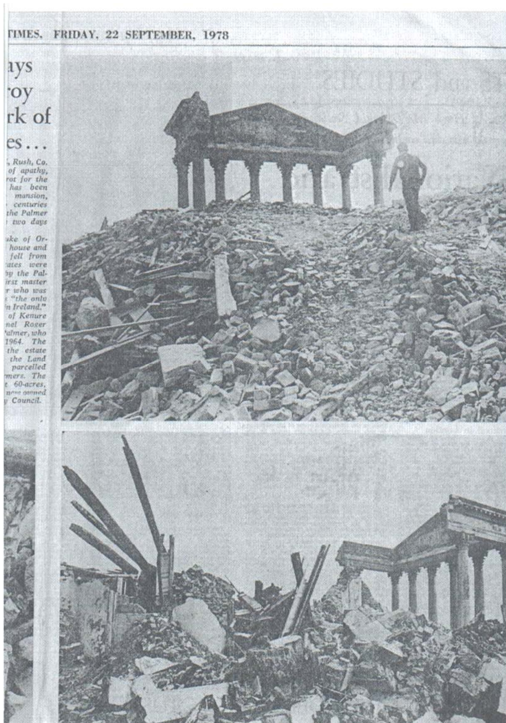
The piles of rubble after the destruction of Kenure House in September, 1978.
