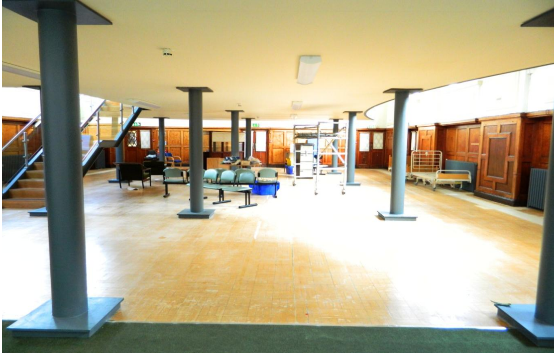
Figure 8.1 – Dining hall of Ardee Mental Hospital: free standing mezzanine level (Photographed by L. Butterly, 2012)
