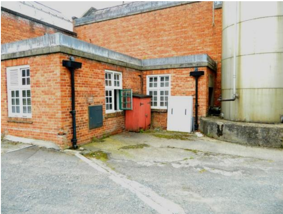
Maintenance building, exterior view, Ardee Mental Hospital (Photographed by L. Butterly, 2012)
