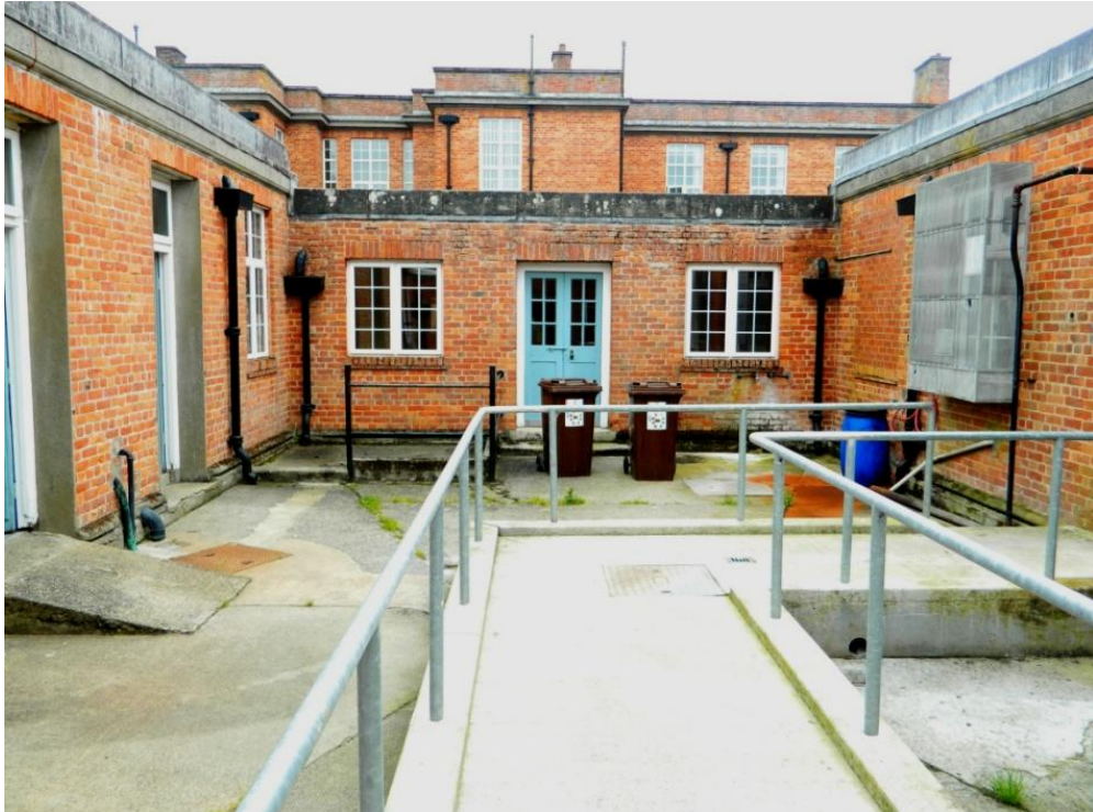
Maintenance area, central block, Ardee Mental Hospital (Photographed by L. Butterly, 2012)
