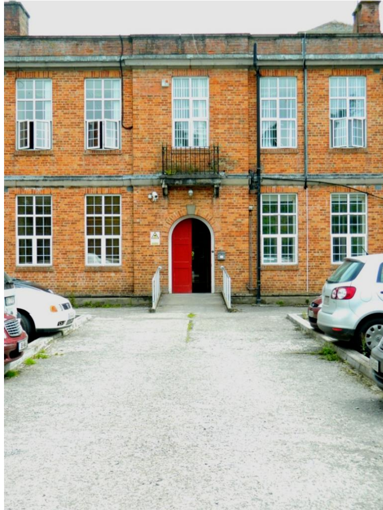
Figure 6.2- Exit door on corridor, Ardee Mental Hospital (Photographed by L. Butterly, 2012)
