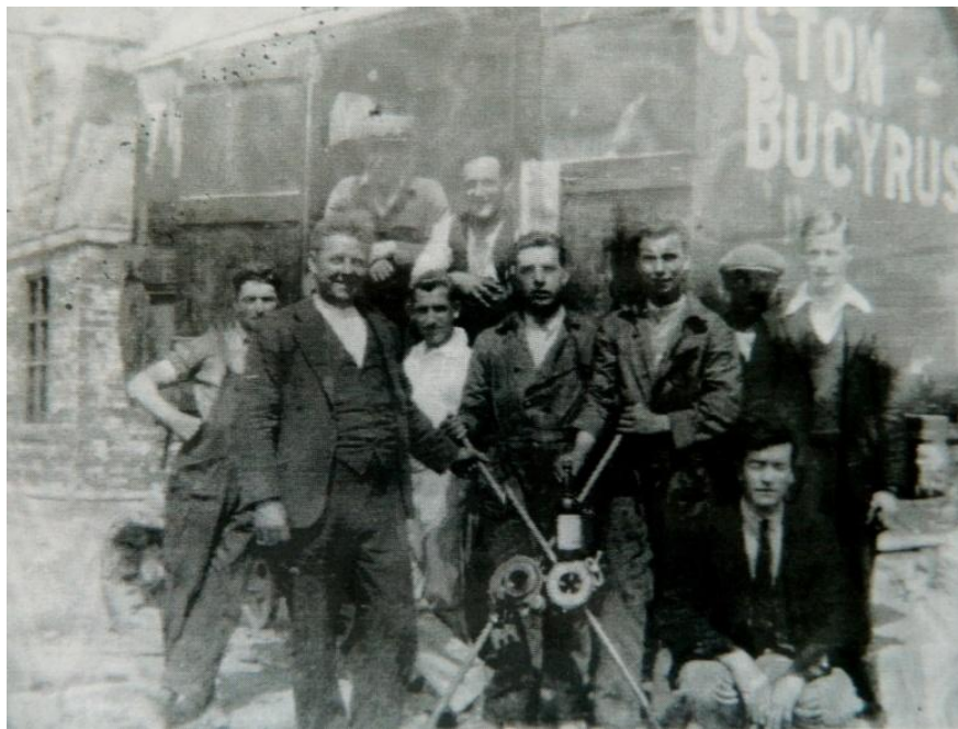
Figure 5.2 – Ruston-Bucyrus excavator photographed on Ardee Mental Hospital site, Dundalk Democrat , 13 Mar. 1932.
