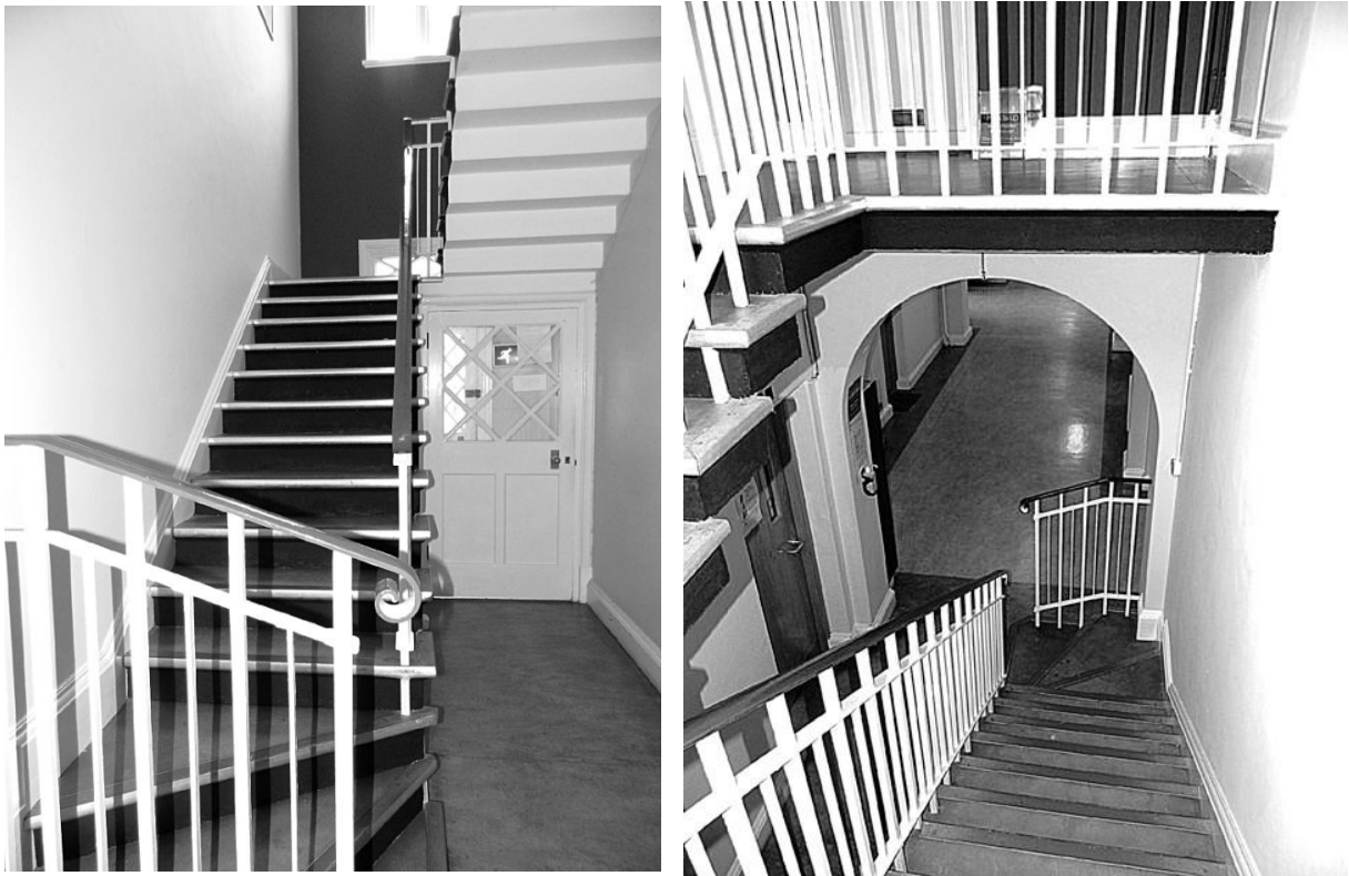
Figure 6.3-4: Staircase, Ardee Mental Hospital (Photographed by L. Butterly, 2012)
