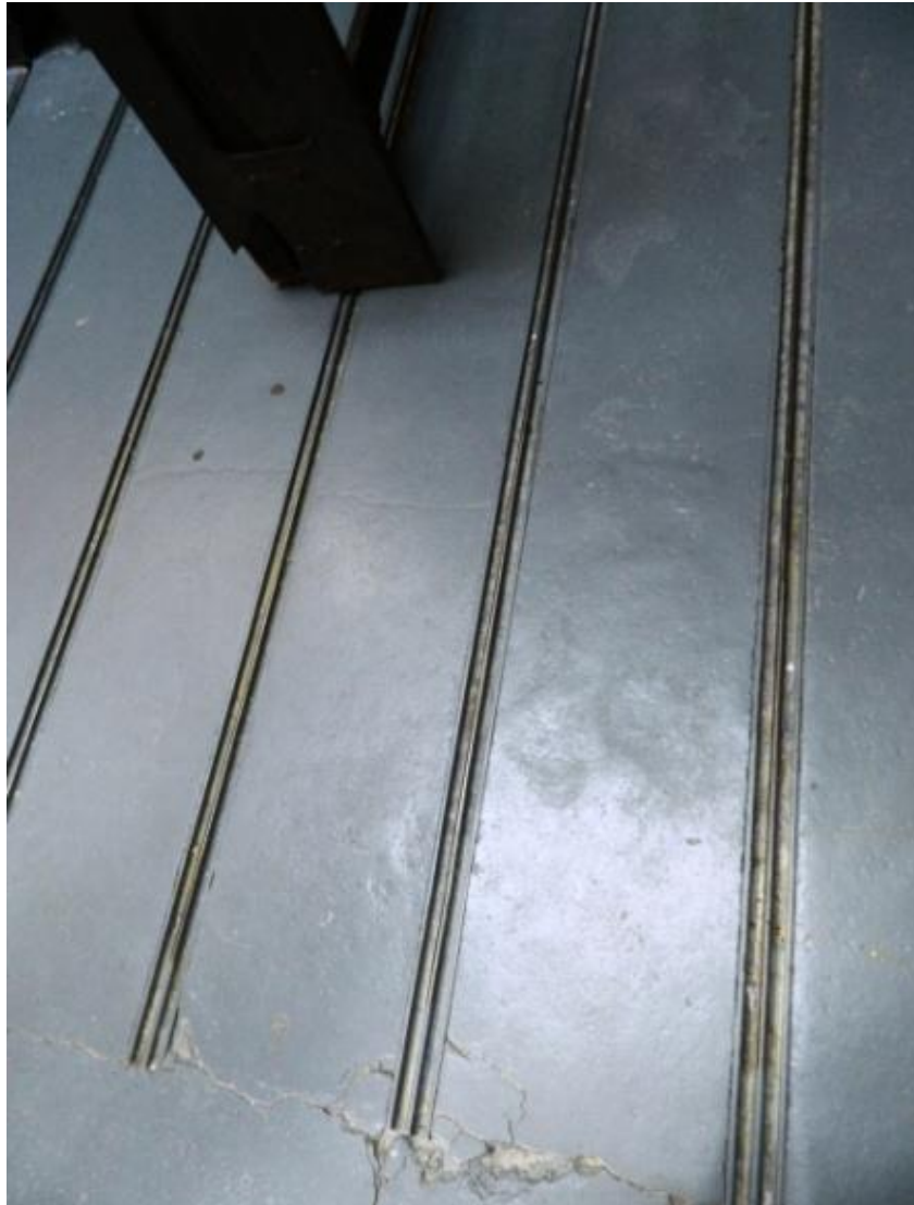
Bradford machinery in laundry building, Ardee Mental Hospital (Floor tracks for rolling shelves) (Photographed by L. Butterly, 2012)
