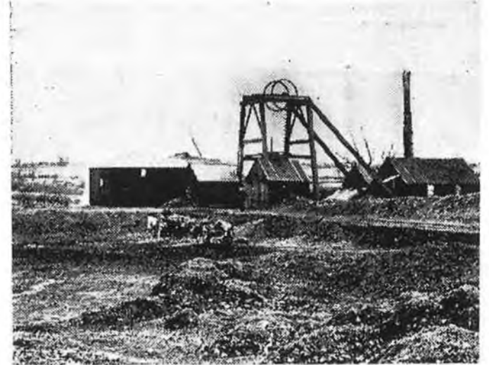
Rock Bog Colliery 1916. Depth of shaft 60 yards. Daily output 40 tons. Total men and boys employed 63.
