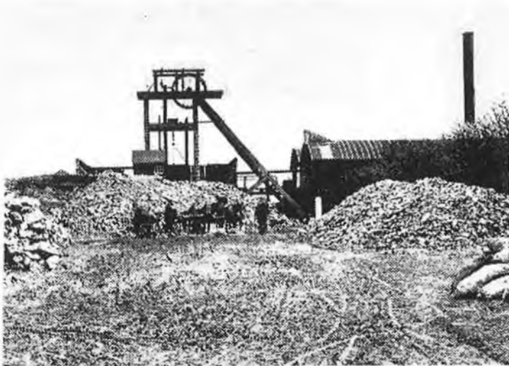
Row Colliery 1916. Depth of shaft 80 yards. Daily output 100 tons. Total men and boys employed 160.
