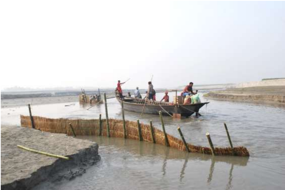
Figure 10: Indigenous engineering for improving navigation at Balashi ghat. Photo by researcher.
