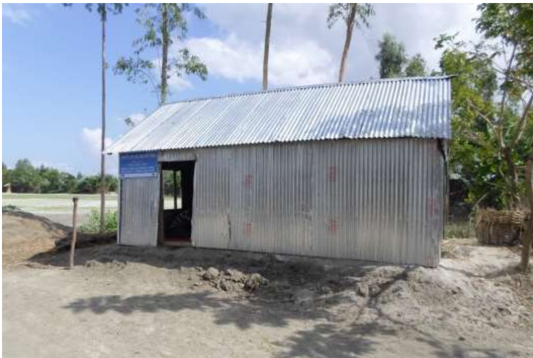
Figure 30: The CBC Office. Photo by researcher.
