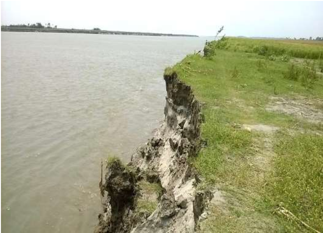
Figure 2: Riverbank erosion. Photo by researcher.
