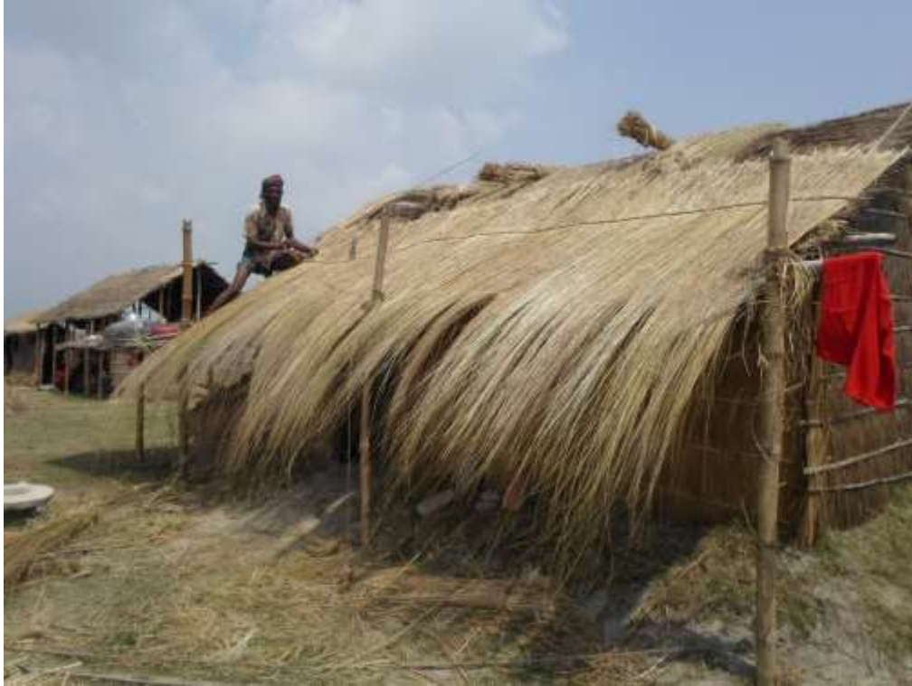
Figure 6: A man rebuilding his house. Photo by researcher.
